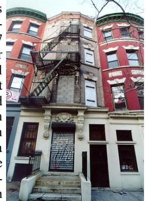
The abandoned Brownstone WE ACT has purchased and will be renovating.
